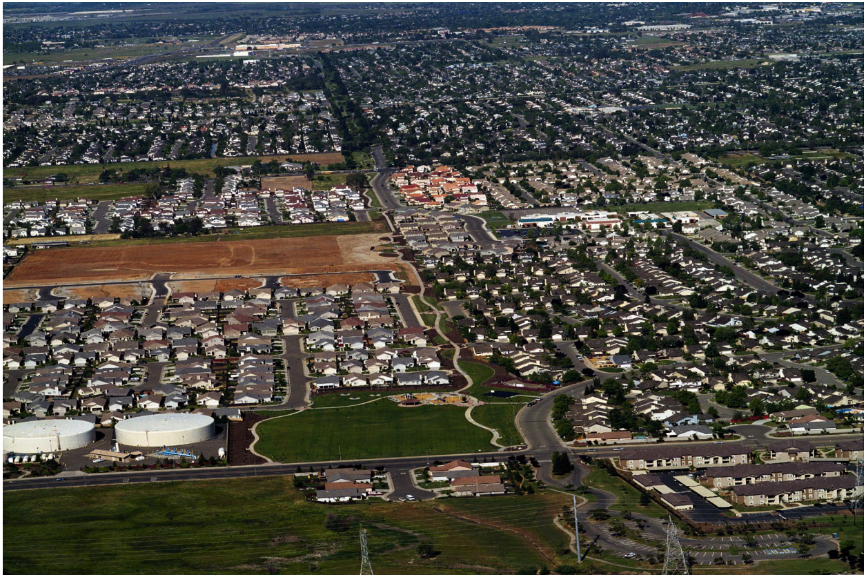
Tillotson Parkway at Boulder Glen Park Under Construction – 2005
